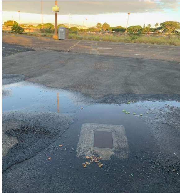
Current Potable water leak in LHPL
