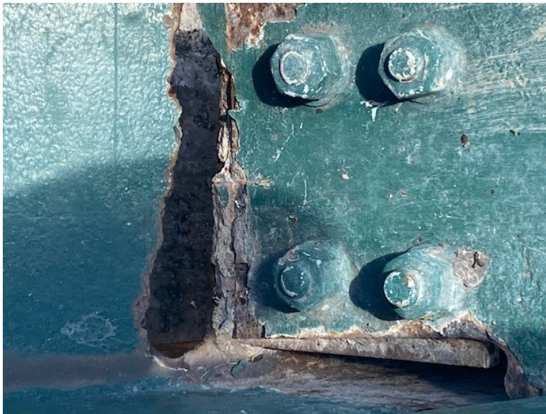
WJE Monitoring – Close-up of corroded diagonal cross brace.
