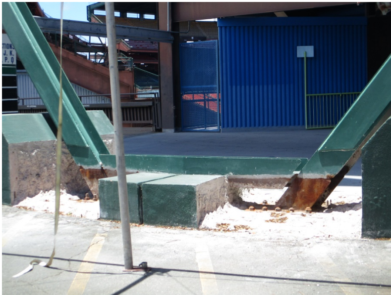
WJE Structural Monitoring – Exposed Brace ready for testing.
