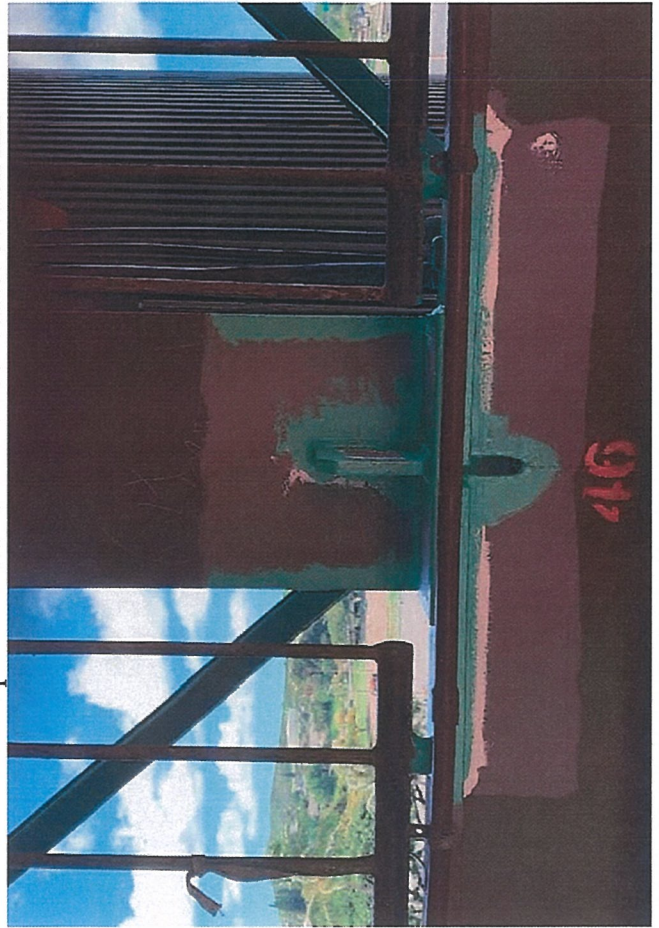
Beam replacement under Inner Concourse Section AA
