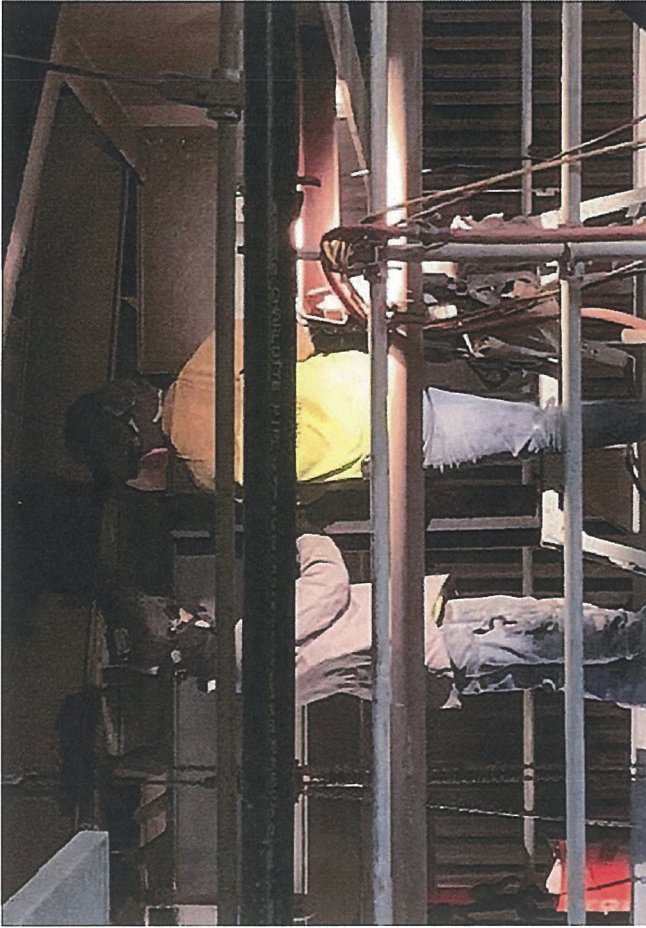
Beam replacement under Inner Concourse Section AA
