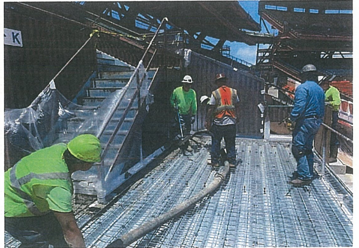
Inner concourse replacement Section K (1)
