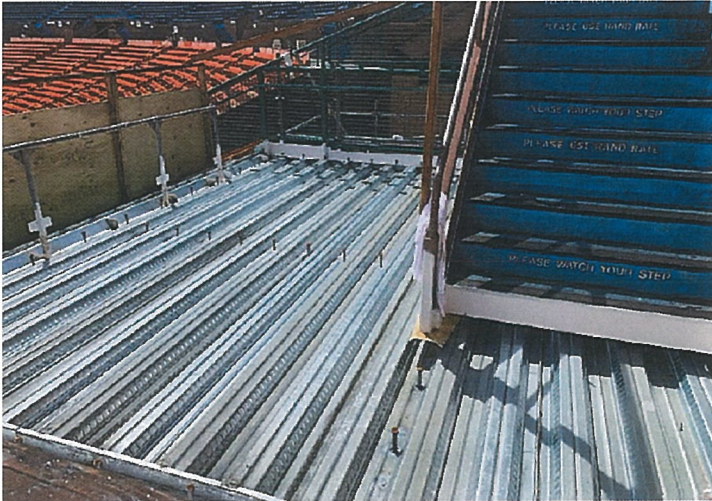
Inner Lower Concourse replacement Sec. F
