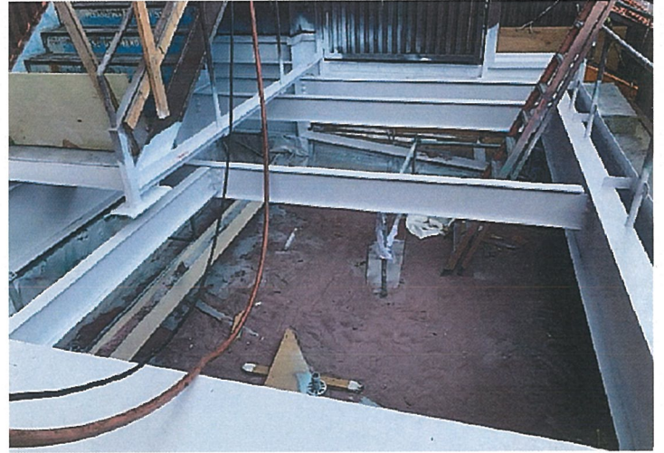
Inner Lower Concourse replacement Sec. K
