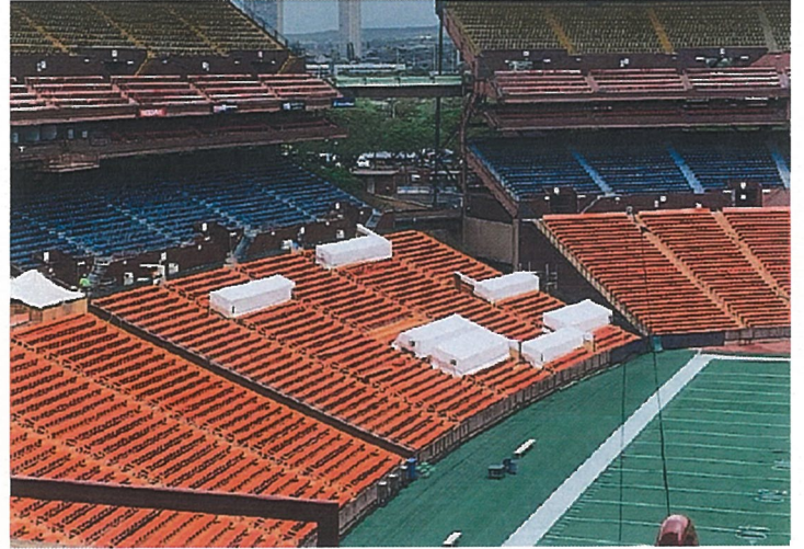
Seat Plate Repairs Orange Section L-Q
