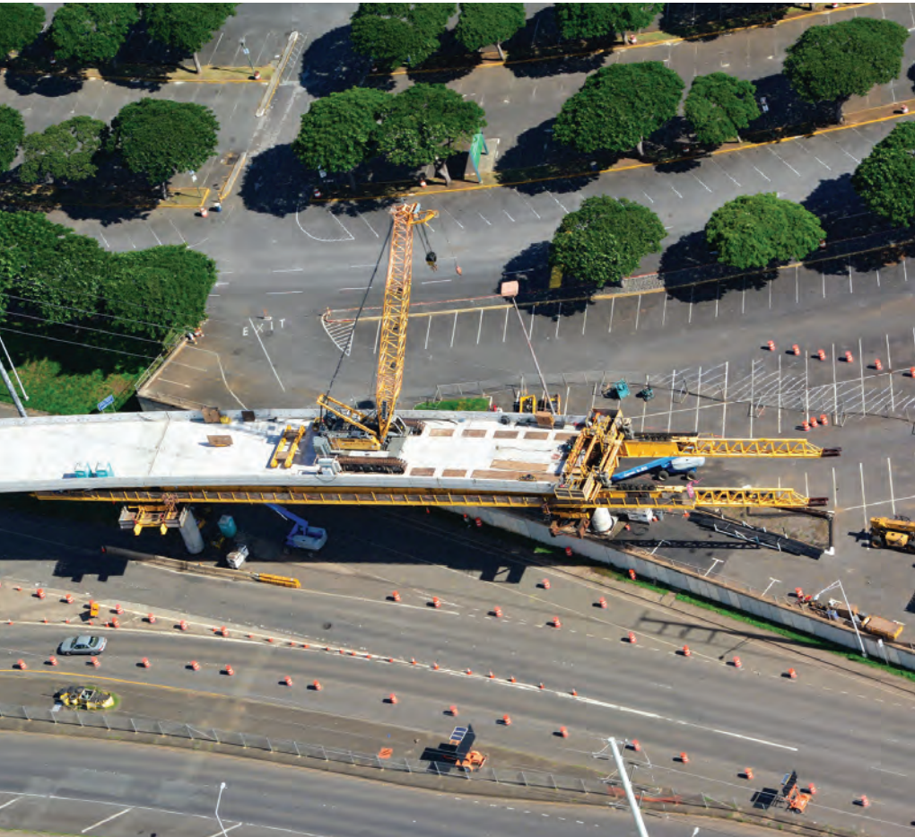
Construction of HART Station
