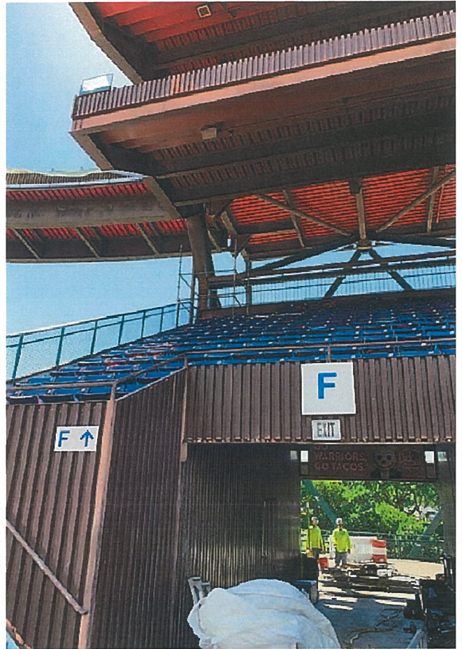
Clip Repair at Top of Blue Level
