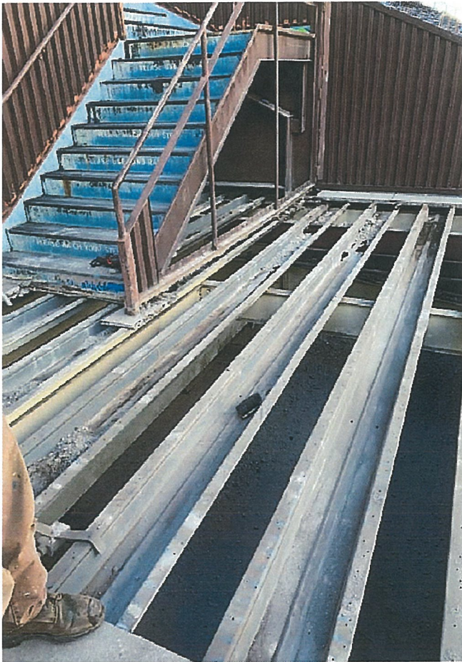
Section K inner concourse repair
