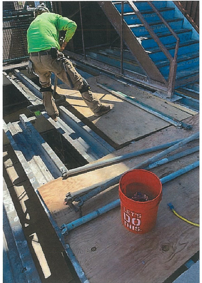
Section F inner concourse repair
