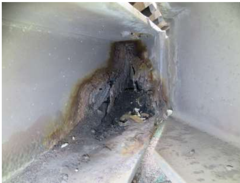
Figure 13. Additional example of structural steel member classified as Condition State 4.
