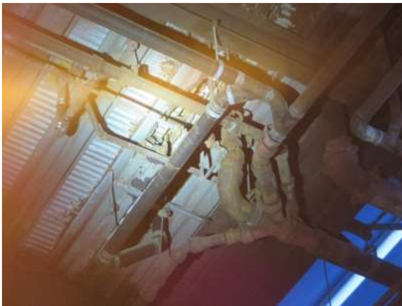
Figure 23. Deteriorated decking and sub-decking at plumbing penetrations servicing a toilet facility in a sideline seating stand.
