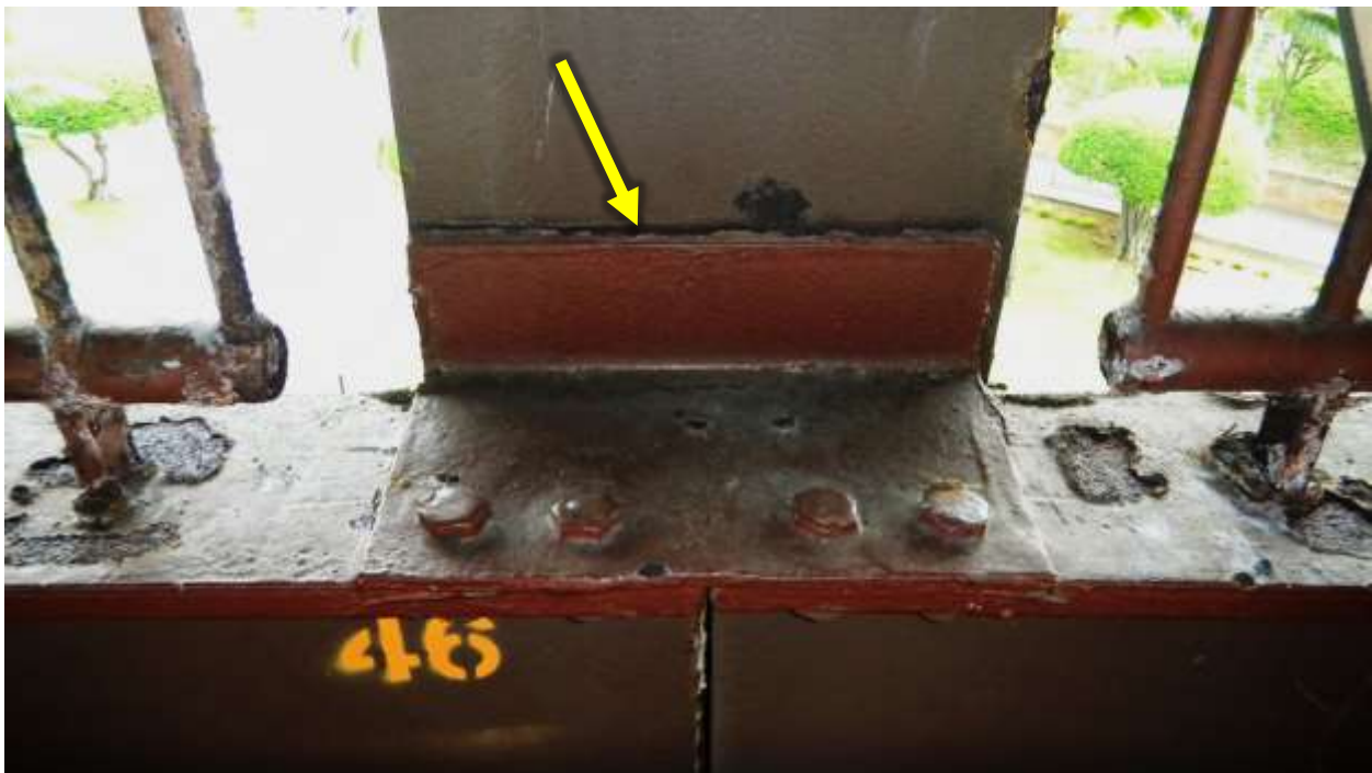
Figure 20. The indicated weld line between connection angle and raker column flange has completely fractured.
