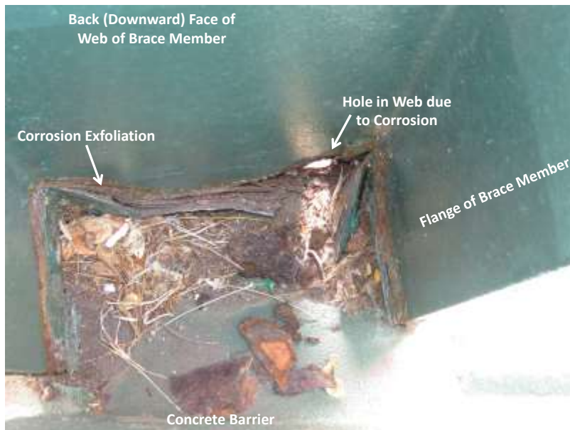
Figure 18. Annotated photo showing severe corrosion conditions at base connection of steel brace member to the concrete barrier (South endzone).
