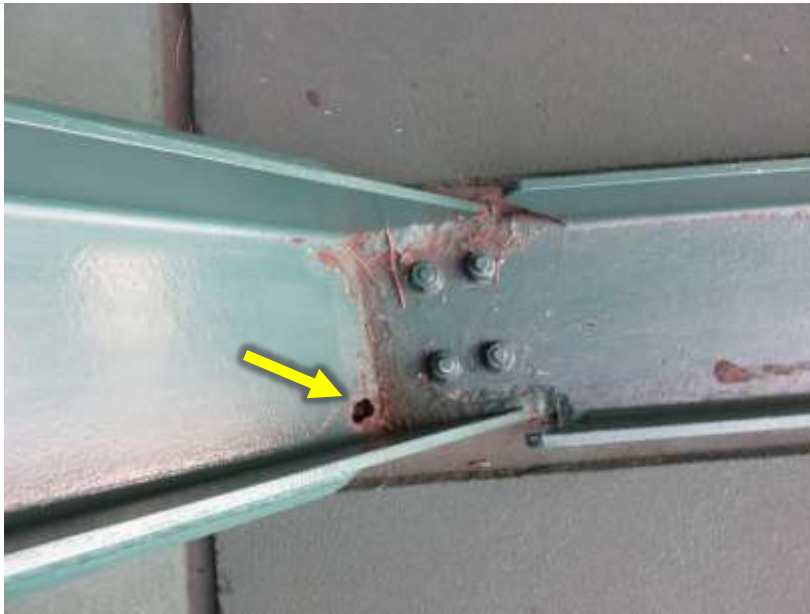
Figure 12. Example of structural steel member classified as Condition State 4. The yellow arrow points to a hole completely corroded through the thickness of the web of the steel member.
