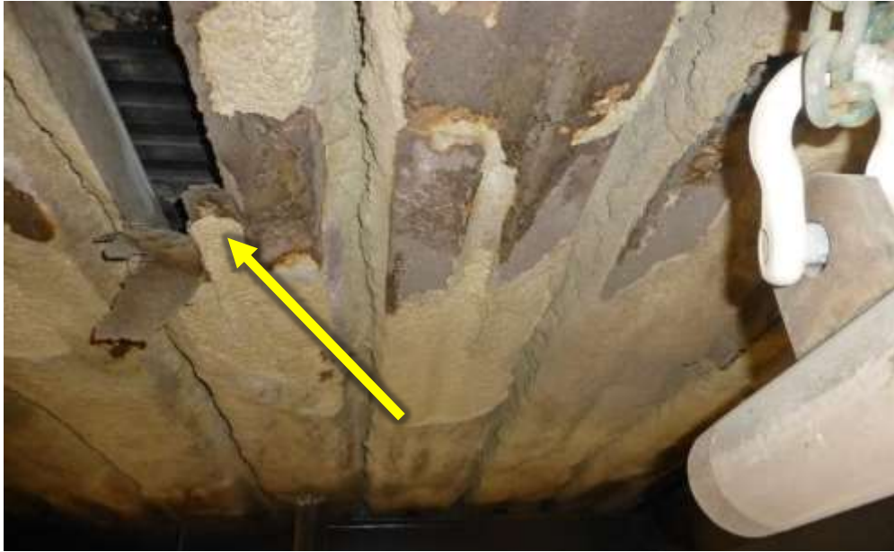
Figure 24. Corrosion has occurred through the lightweight sub-decking hat channel that supports an electrical room floor at the Northeast Sideline seating stand.
