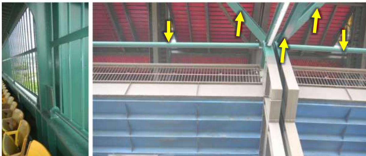
Figure 8. Examples of structural steel members classified as Condition State 1
