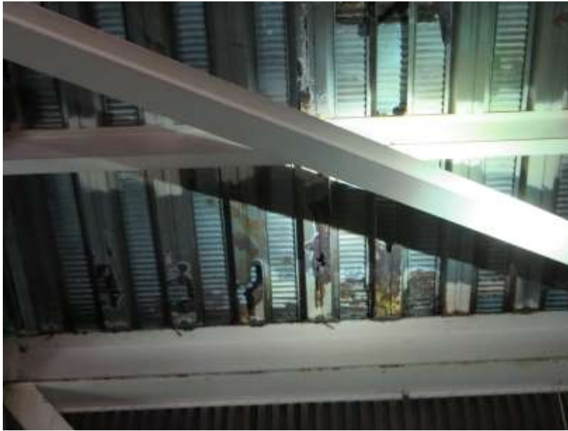
Figure 22. Representative severe (CS4) corrosion conditions observed in decking and hat-channel sub-decking of the lightweight floor system of the lower concourse of a sideline seating stands. Location shown is where the decking is supported by the end bay radial truss (at bottom of photo) of the sideline seating stand.
