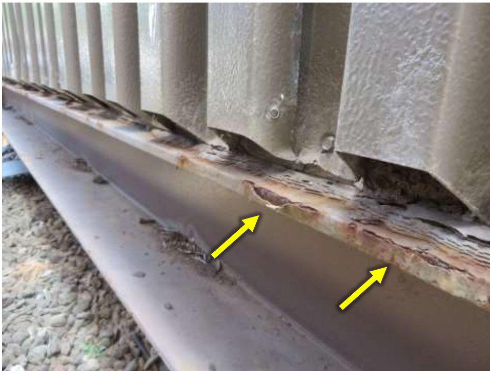
Figure 10. Example of structural steel member classified as Condition State 3.
