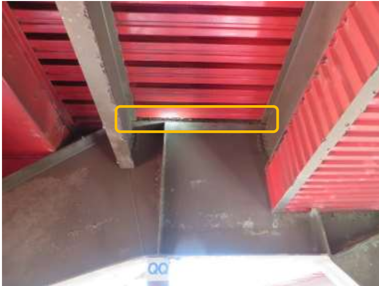
Figure 16. Corroding top flange of deep raker beam supporting the Red seating area. This location is in an end frame of the northeast sideline stands. The deep beam is one component of the cantilever raker assembly that supports the Red and Brown seating areas.
