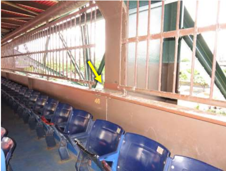
Figure 19. Typical location of problematic Blue seating section connection between girder and raker frame column.
