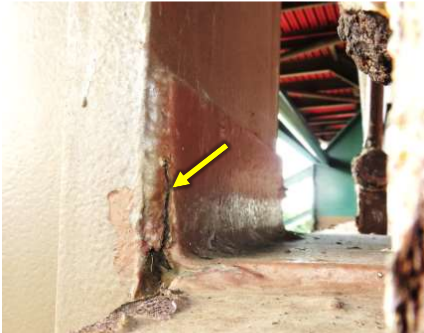
Figure 21. The weld between the connection angle and raker column flange at this location has partially fractured.
