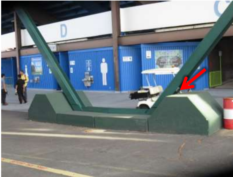
Figure 17. Representative concrete barrier at base of structural steel braces that make up the diagonal bracing frame at the rear of the endzone seating stands (South endzone shown). The red arrow indicates viewing position for the photo of Figure 18.
