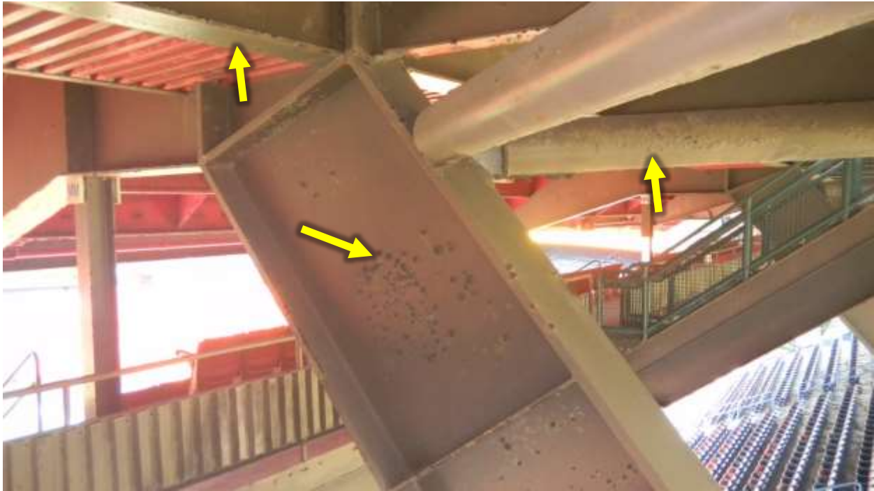
Figure 9. Example of structural steel member classified as Condition State 2
