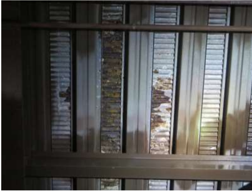
Figure 11. Example of lightweight floor slab decking classified as Condition State 3.
