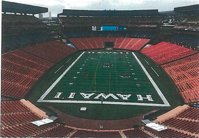
Mauka and Makai Orange Section Rehab Complete
