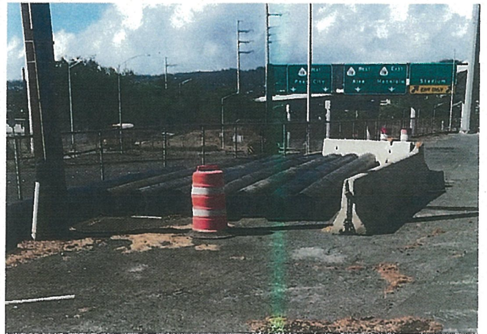
Removal of Force Main Bypass Pipe
