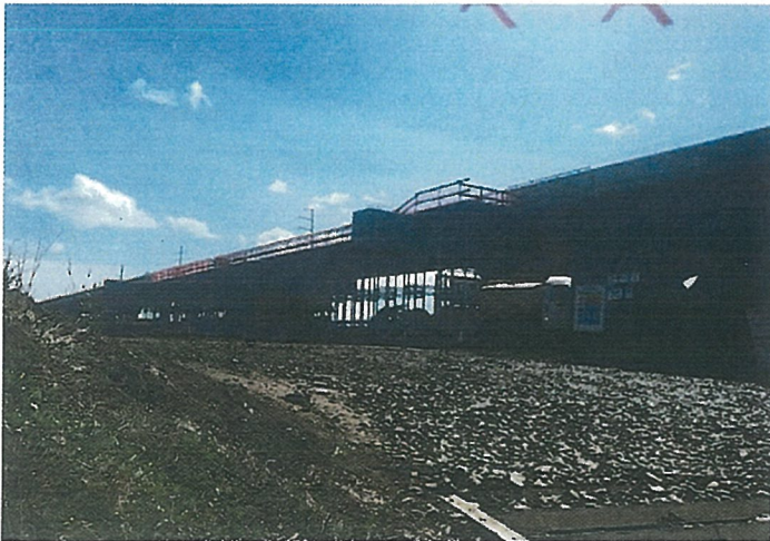
Scaffolding for AS HART Station
