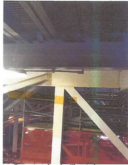
Beam staged under Electrical room
