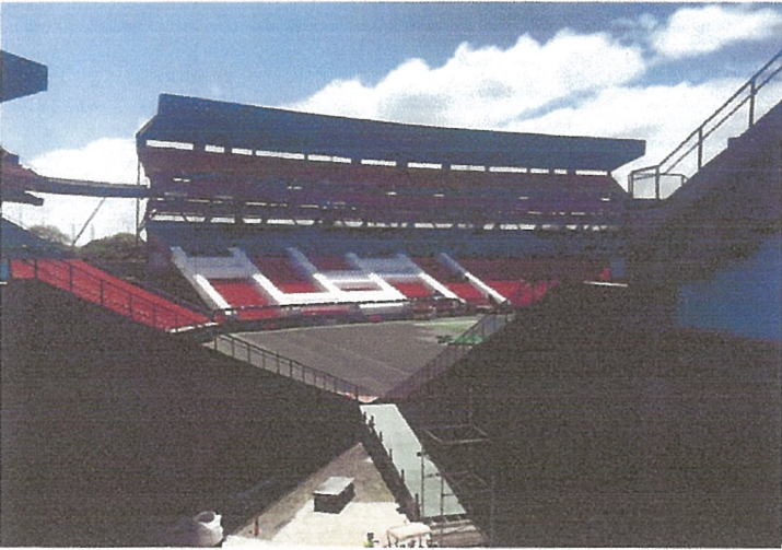
Makai Side under repair
