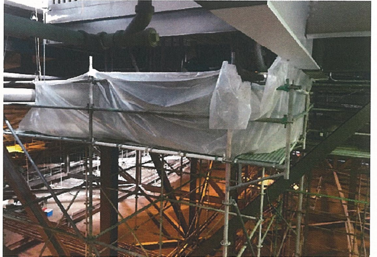
Removal of Fireproofing under MM Electrical Room (Non-Asbestos)
