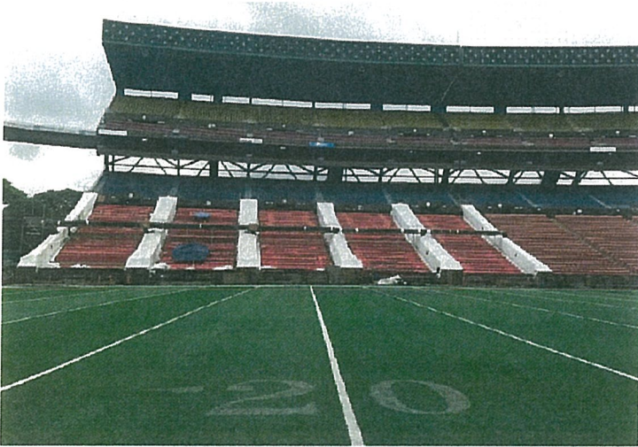
Section LL-QQ seat plate repairs
