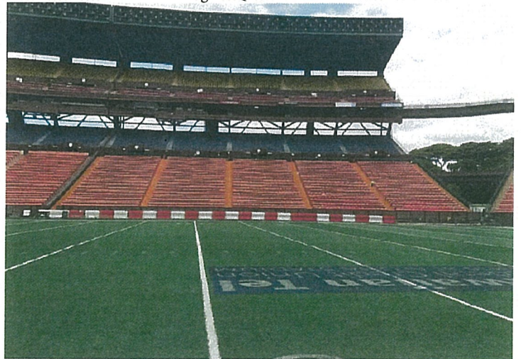
Orange Section L-Q Completed
